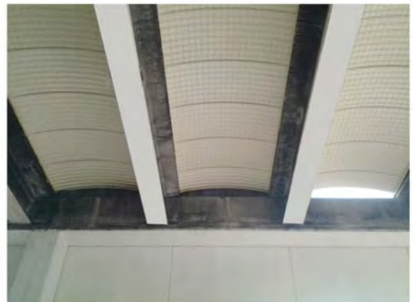
CONSTRUCTION OF CURVED ROOF BY NOTCHING OF ITP MONO28
